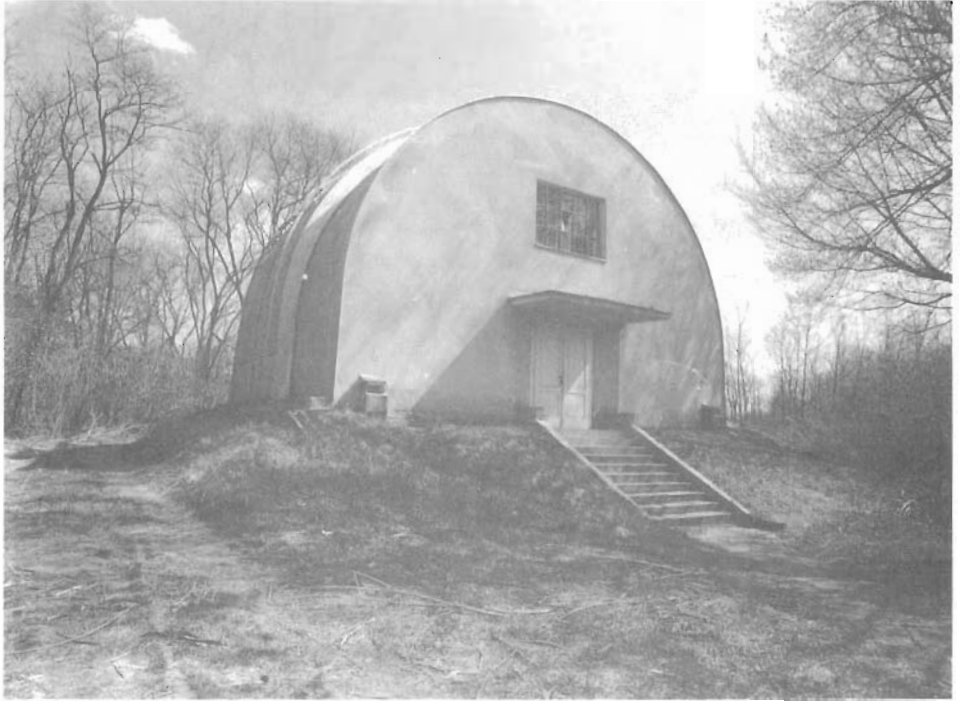
Fig. 15. The pavilion of the Large Meridian Circle "Ascania".
